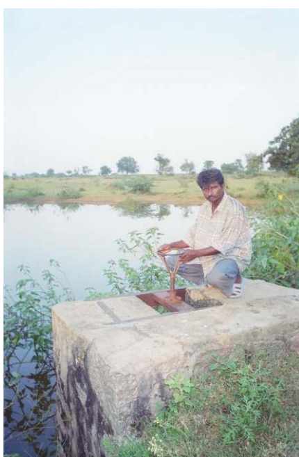
Regulation of tank water by Nirdee
