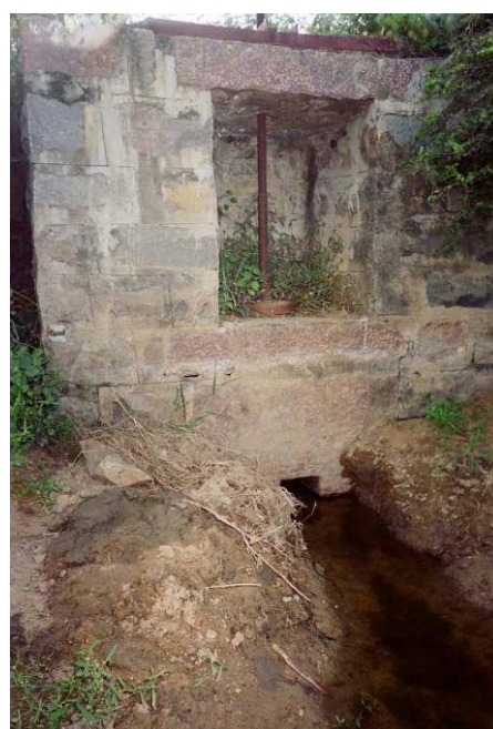
Spindle and rod mechanism of the outlet
