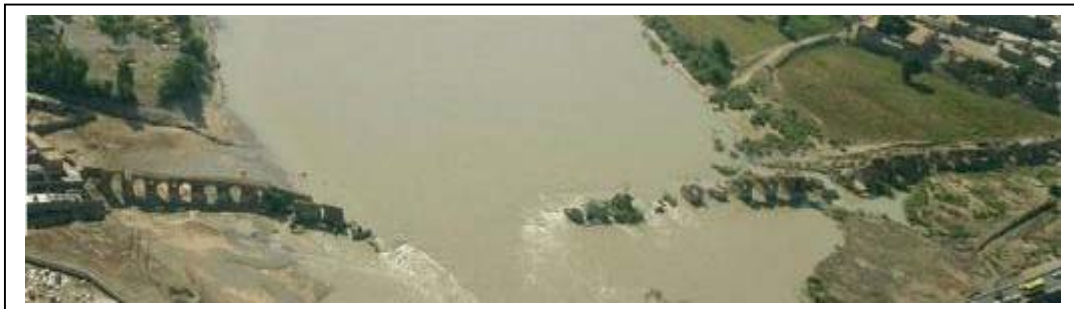
Fig (3) – Shadravan barrier- bridge
