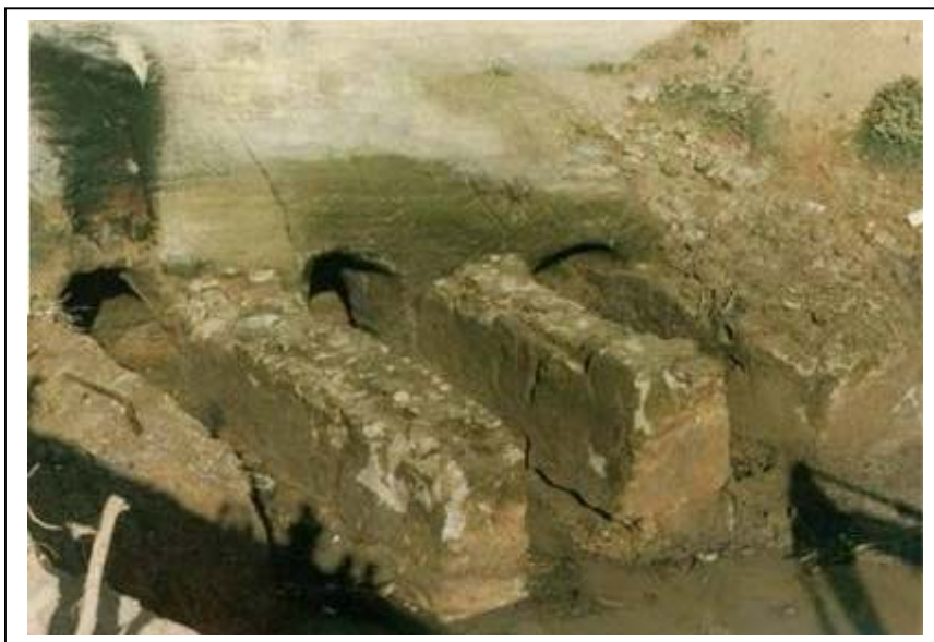
Fig (5)- Three – Coreh tunnel inlet.
