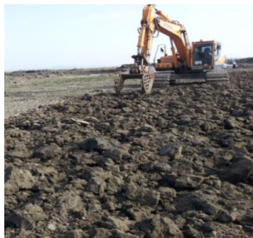
Image 1. Subsoil Breaking Using A Backhoe
