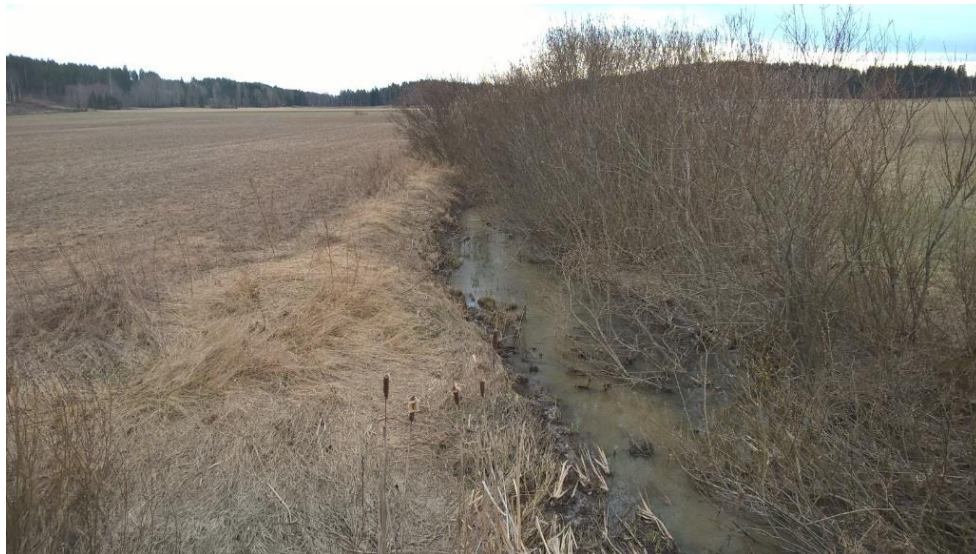
Figure 7 (Elsi Kauppinen). Mättäänoja-ditch in April 2016, before growth season. Low drainage depth is causing the fields to have regular flooding after snow melt and heavy rains.
