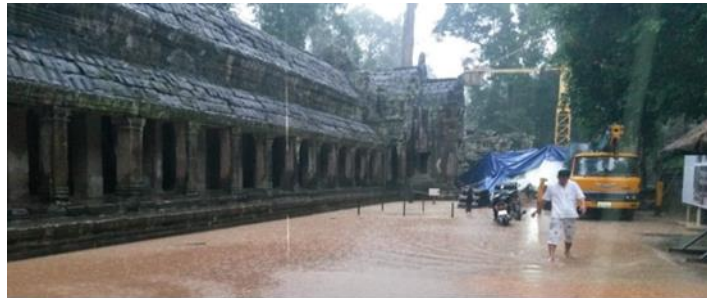
Figure 3: Water Stagnation between Third & Second enclosure
