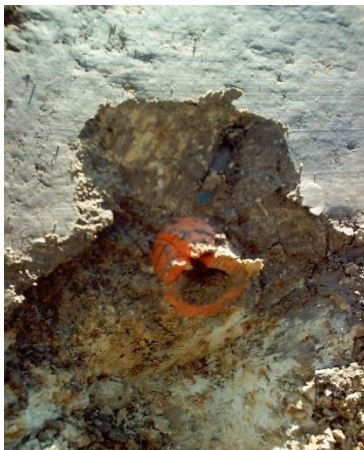
Picture 3. Silty clay drainage pipe
