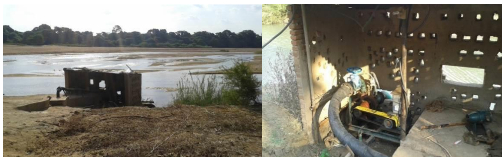
Figure 11. Pump plinth for Vimbanayi & Zuvarabuda constructed near the river bank
