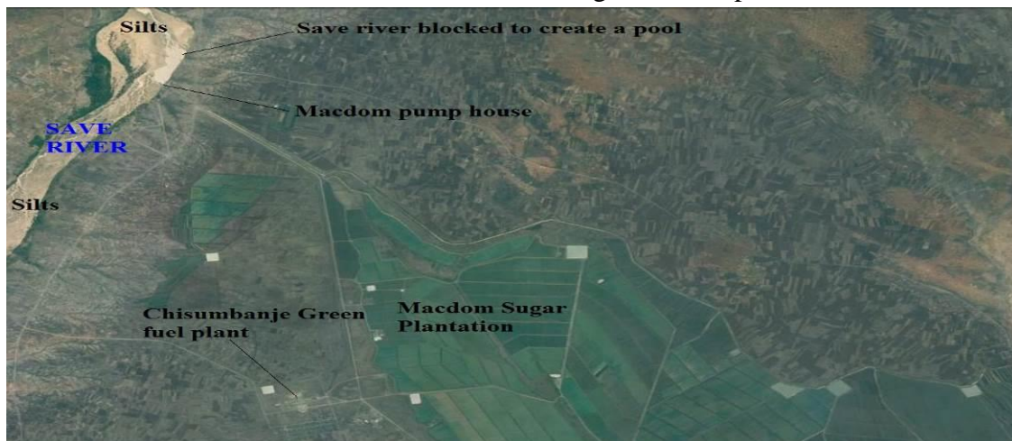
Figure 7. The Save River blocked to create a pool around the Macdom pump house
