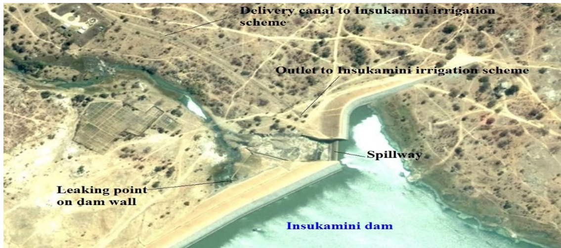
Figure 6. Insukamini leaking dam wall
