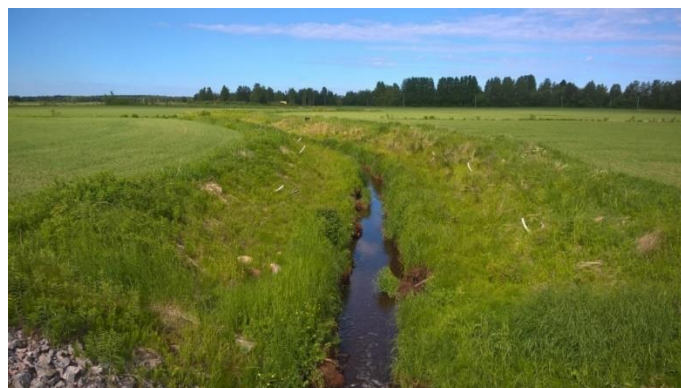
Figure 5 (Elsi Kauppinen). Two-stage drainage channel at Leppioja, a few years after construction work. Connections to subsurface drains for easier flushing are visible on the sides.
