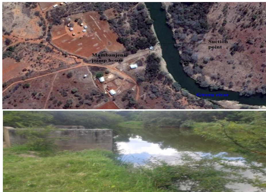
Figure 12 Plinth and pump house at Mambanjeni built on the river bank
