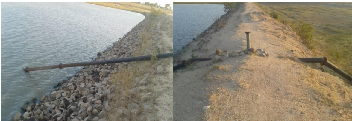
Figure 5. The syphoning system of water abstraction at Mutorahuku dam in Sept. 2014
