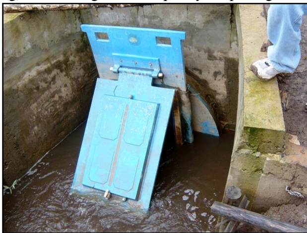
Figure 6. Prototype model and operation principle of double functioned fiber glass flap gate (left); Figure 7. Flap gates installed at hydraulic structure for operation (right)
