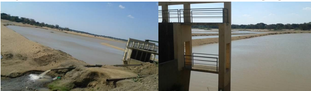
Figure 8. The Save River completely blocked at the Macdom pump house a week after the onset of the rainy season in November 2014
