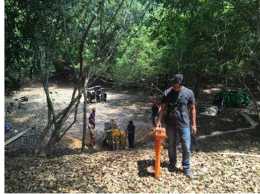
Figure 10: Detection of Drilling tool path by Directional Probe & Magnetic Field Locator
