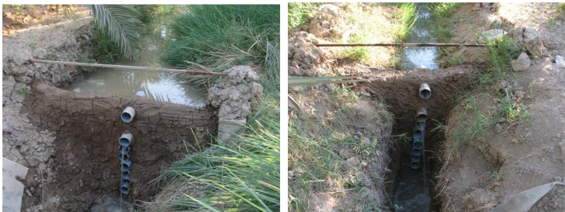
Figure 6. Small water tight dams at lower ends of the drain ditches
