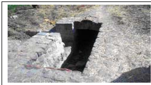
Photo 4: Transformation from Underground Channel to Open Channel
