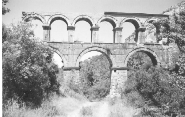
Figure–2: Sextilius Pollio aqueduct over Marnas Valley.
