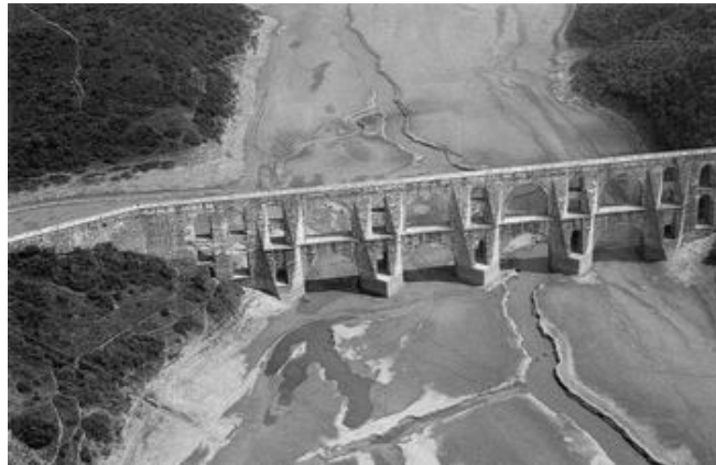
Figure–5: Maglova (Muglava) aqueduct with 35 m height and 258 m length was constructed by Architect Sinan on the Kirkcesme water conveyance system (Cecen, 1996).
