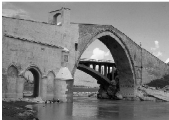
Figure–4: Malabadi Bridge with a 39 m single span width.
