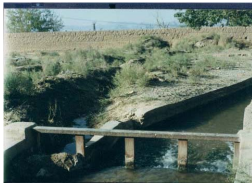
Figure 1- a traditional structure named Maqdam for dividing water into four shares each of which goes to a particular village. (the province of Yazd)
