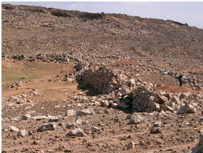
Figure 1: The old dam at Jawa
