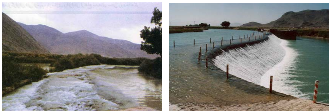
Figure3. Feizabad dam before and after rehabilitation
