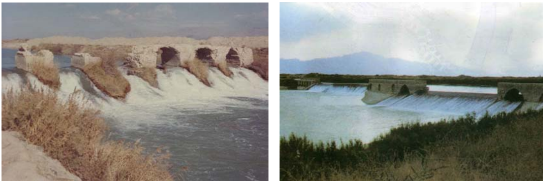
Figure5. Tilakan dam before and after rehabilitation
