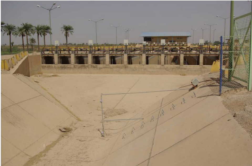
Fig. 3. Silt settlement tanks
