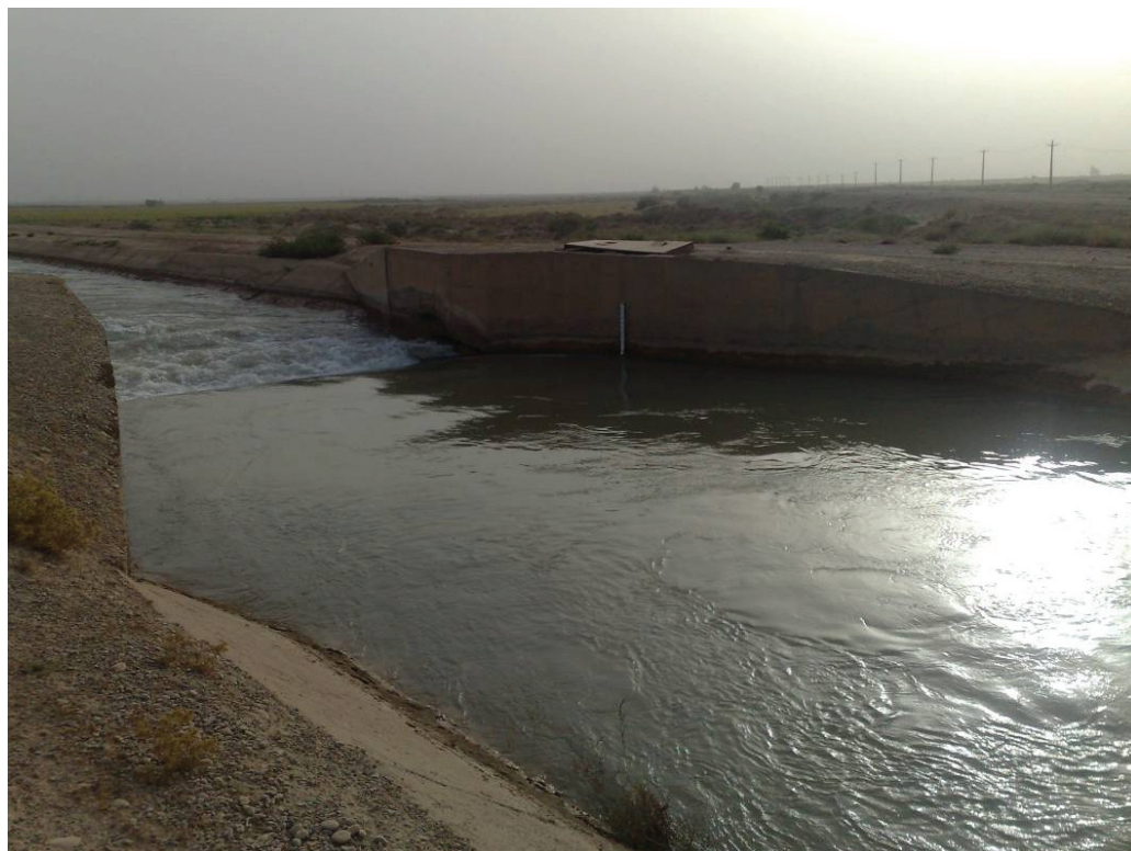
Fig. 5. Parshall flume
