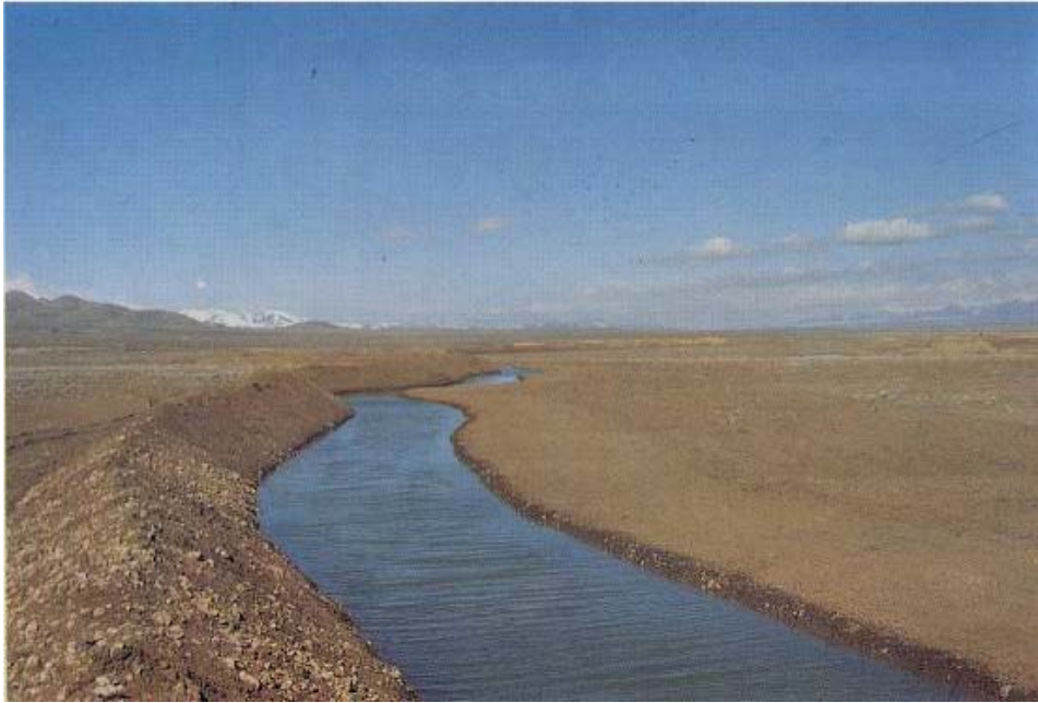
Photo 4: floodwater spreading on aquifers project.
