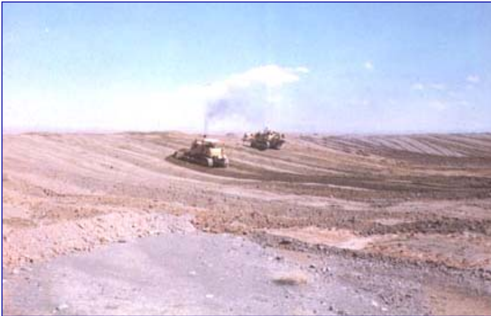
Photo 2: floodwater spreading for artificial recharge of groundwater
