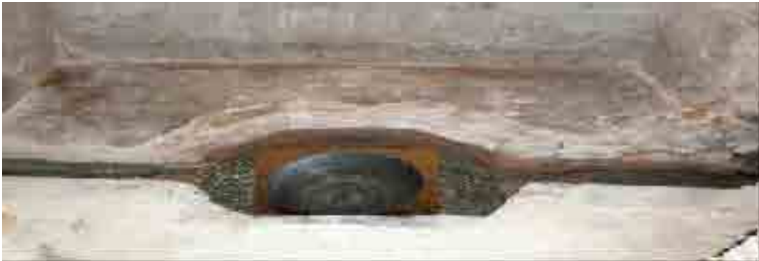
Figure 8: Water allocation system using a bowl with orifice to distribute water between farmers.
