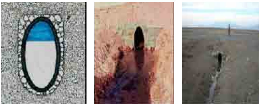
Figure 4. Kouhpayeh tunnel walls have been strengthened with tile hoops in downhill end.
