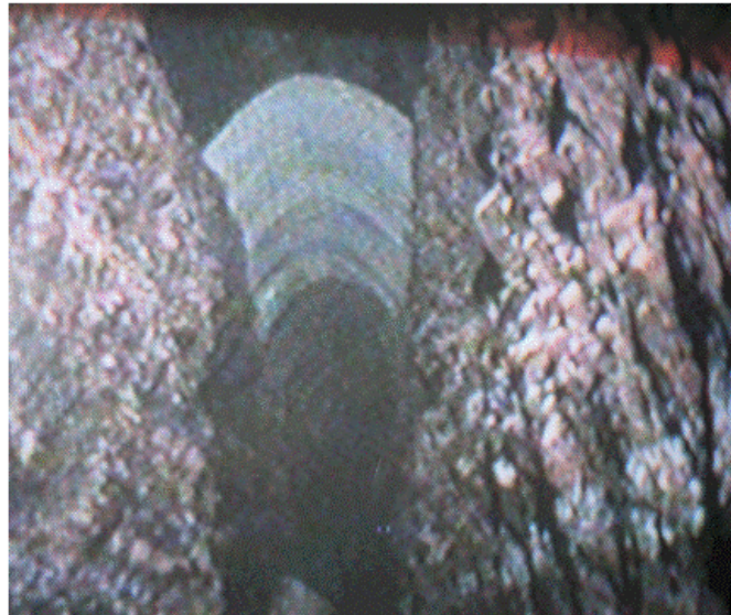
Figure 5 Second ceiling of Vazvan Qanat under construction
