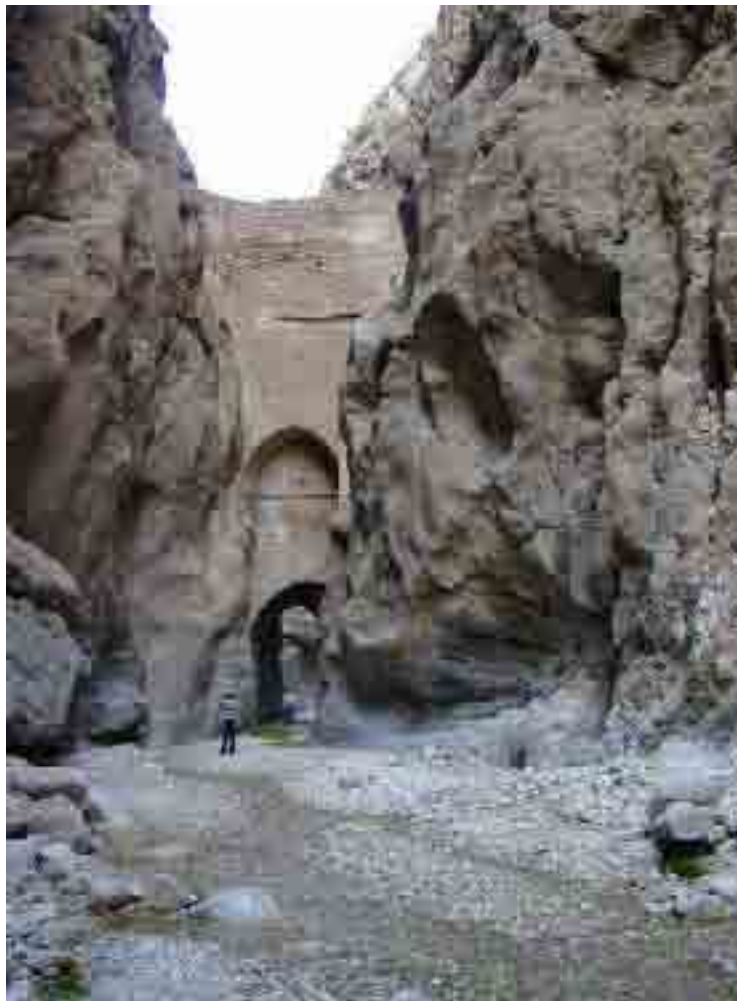
Figure (7) 25 m high Abbasi flood-retarding dam
