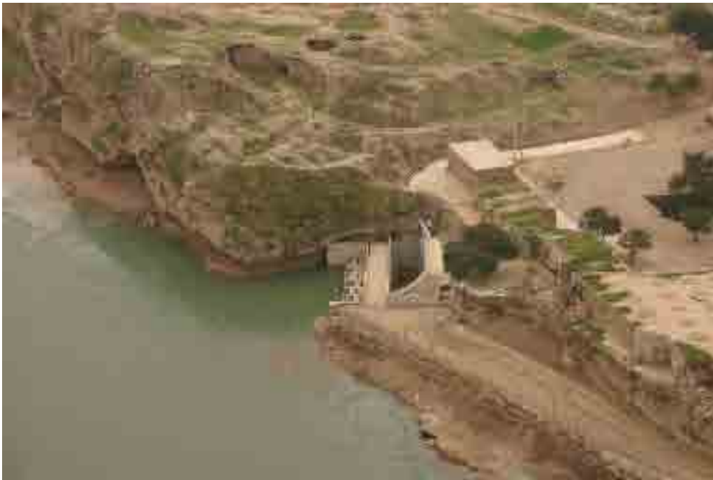
Figure 8. Salasel castle above the turn out of Dariun creek
