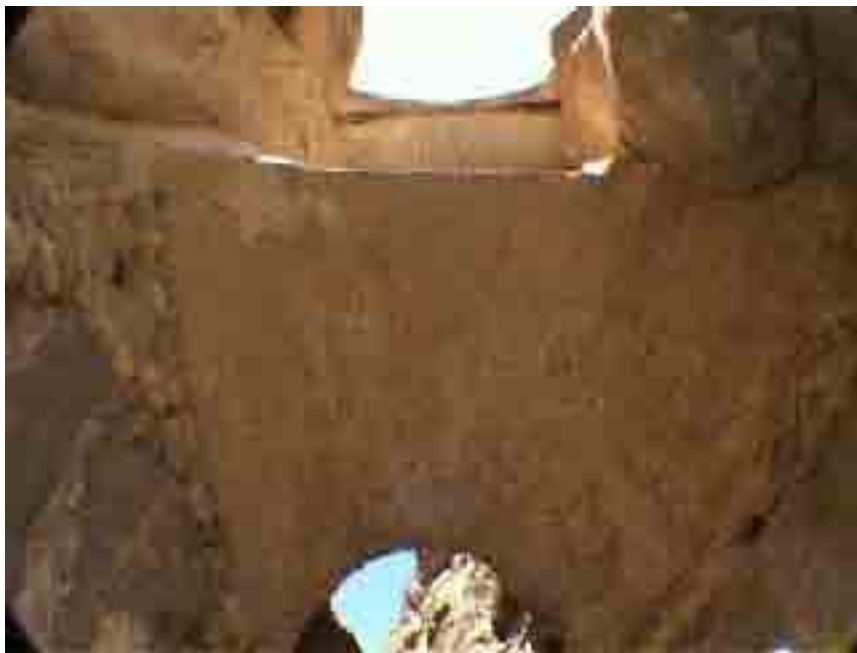
Figure (10). A view of the arch of Abbasi dam from underneath
