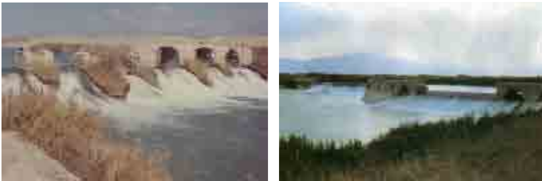
Figure5. Tilakan dam before and after rehabilitation
