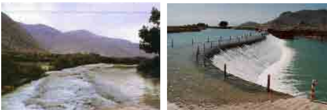
Figure3. Feizabad dam before and after rehabilitation
