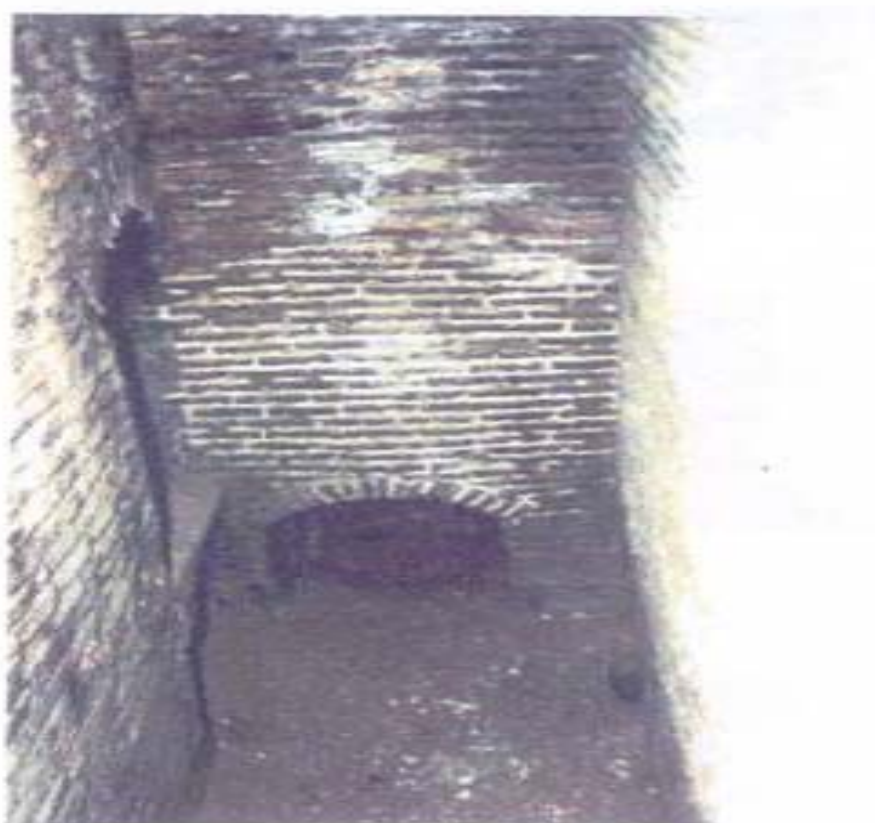
Figure 4. water way of Yagmaey reservoir in Shahrood
