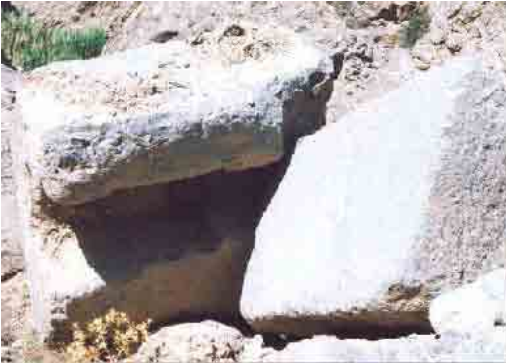
Figure 16. Pieces of U-shape stones making a water conveying small canal downstream of Didegan dam.
