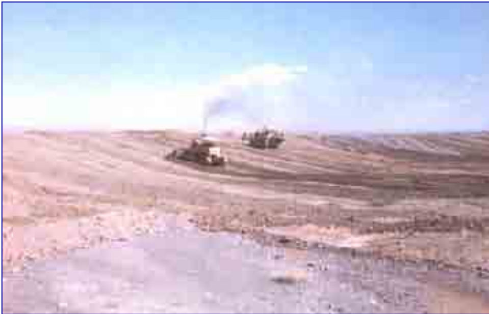
Photo 2: floodwater spreading for artificial recharge of groundwater
