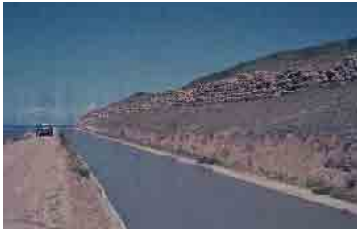
Figure 4: The modern Menua-canal. Above it at the slope the retaining walls of the old structure can be seen (Foto: Garbrecht)
