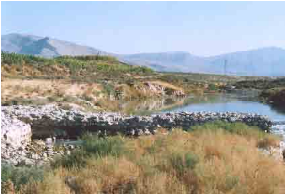
Figure 6. A typical stone masonry diversion dam of the city of Istakhr.
