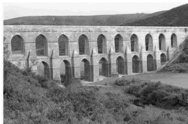
Figure–6: Guzelce (Gozluce) aqueduct with 32 m height and 165 m length was constructed by Architect Sinan on the Kırkcesme water conveyance system (Cecen, 1996).
