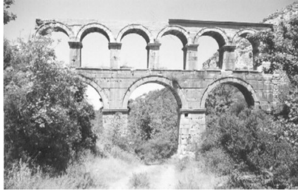
Figure–2: Sextilius Pollio aqueduct over Marnas Valley.
