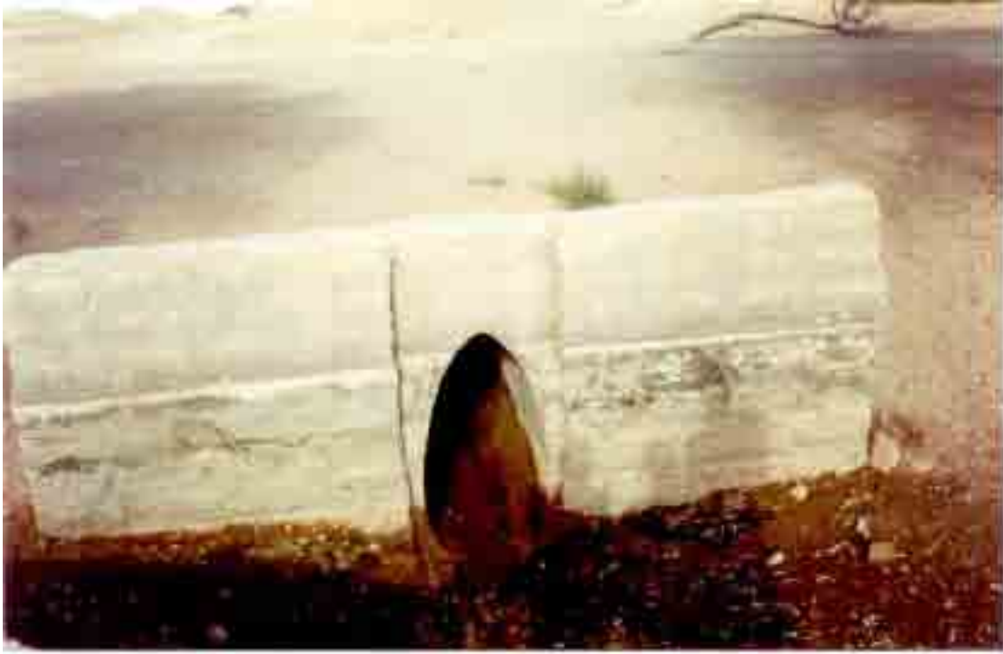
Figure1: Subterranean canal appearance
