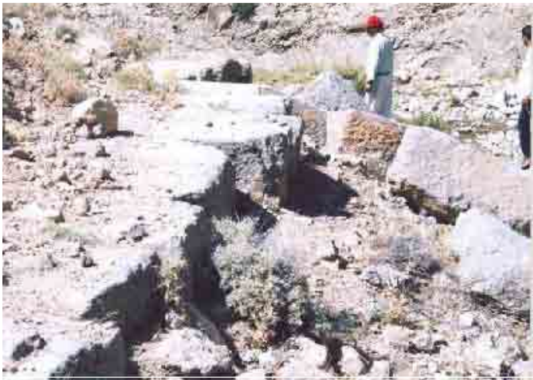
Figure 15. The remaining of stone pavement downstream of Didegan dam. Probably for scour protection.
