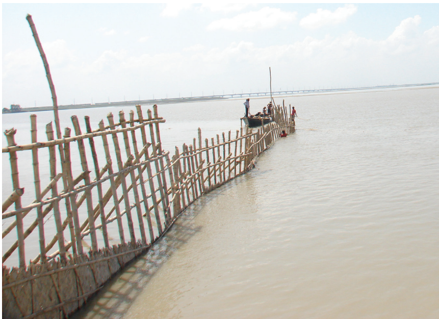
Fig. 3. Bamboo Bandalling in progress in the Jamuna River of Bangladesh
