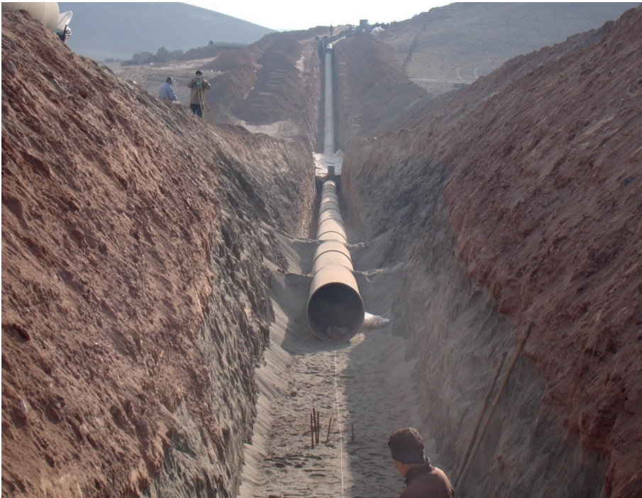
Fig. 4. Inverted Siphon used in Conveyance Canal
