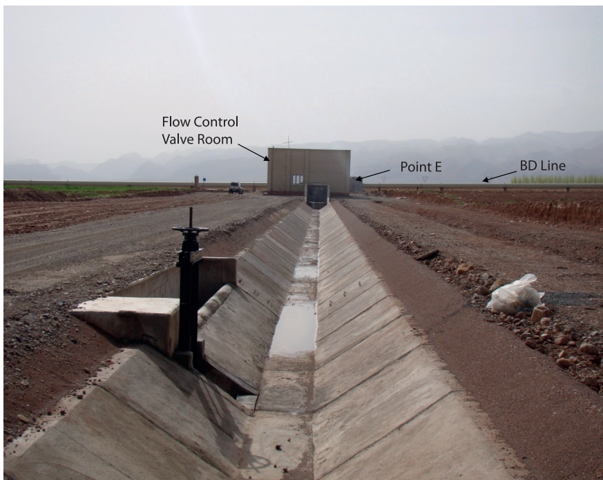
Fig. 2. Flow Control Valve Room, Conveyance Canal and BD Line
